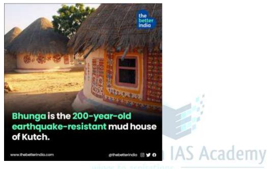
Designed by the people of Kutch in Gujarat after the devastating 1819 earthquake, these circular walled houses have thatched roofs and thick walls made using clay mixed with the dung of cows or camels.
